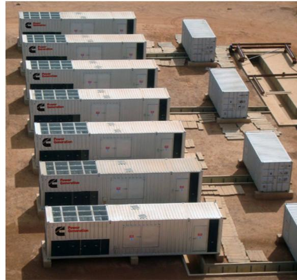
**Figure 3:** Cummins Power Generation generators in climate-controlled enclosures provide power for a gold mine in West Africa.
