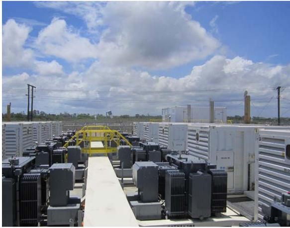
30 x 1000 kW C1250 D2R generator sets provide prime power
