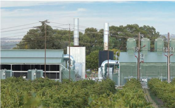
50 MW power plant featuring 30 Cummins QSK60 diesel generator sets located in South Australia to help support the Australian power grid during times of high peak demand or power emergencies.
